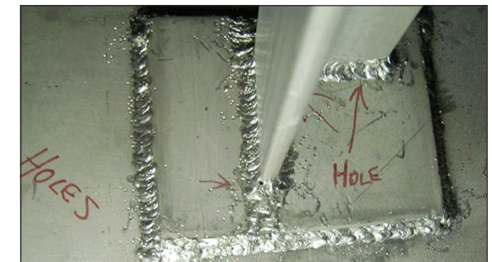
Figure 7. Bioreactor internal welds displaying defects.
