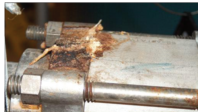
Figure 5. A leaking dextrose hand valve.
