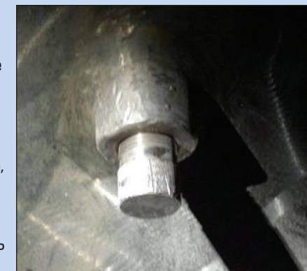
Figure 6. Leaking internal threaded connection in legacy fermentor.
