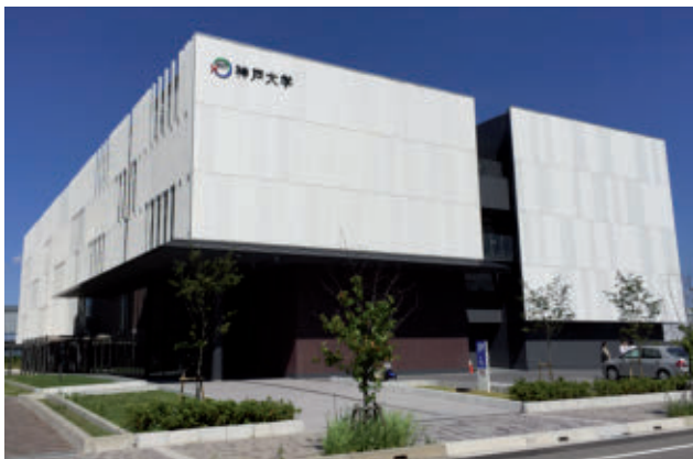
Kobe GMP manufacturing site.
