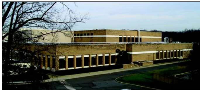
BMS CSO/DPTC facility.
