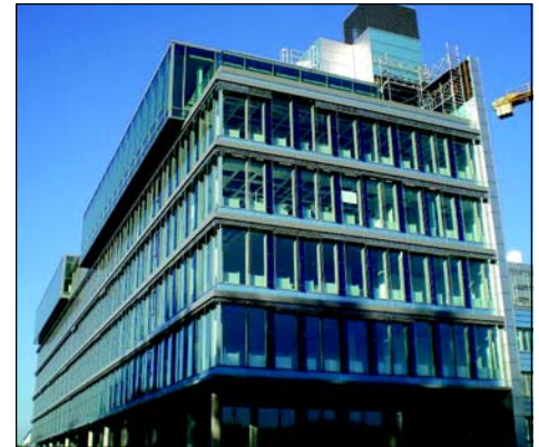
Biologics IV office and laboratory building.
