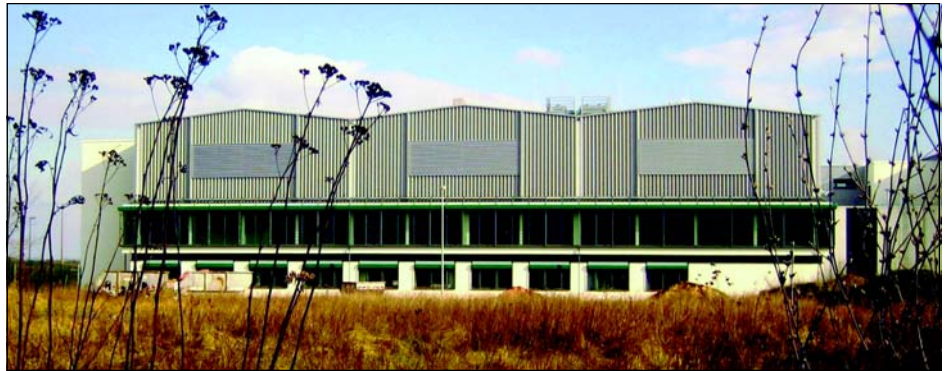
Exterior view on the west side of the new facility.
