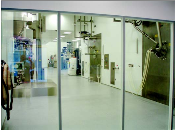
Single containment module.
